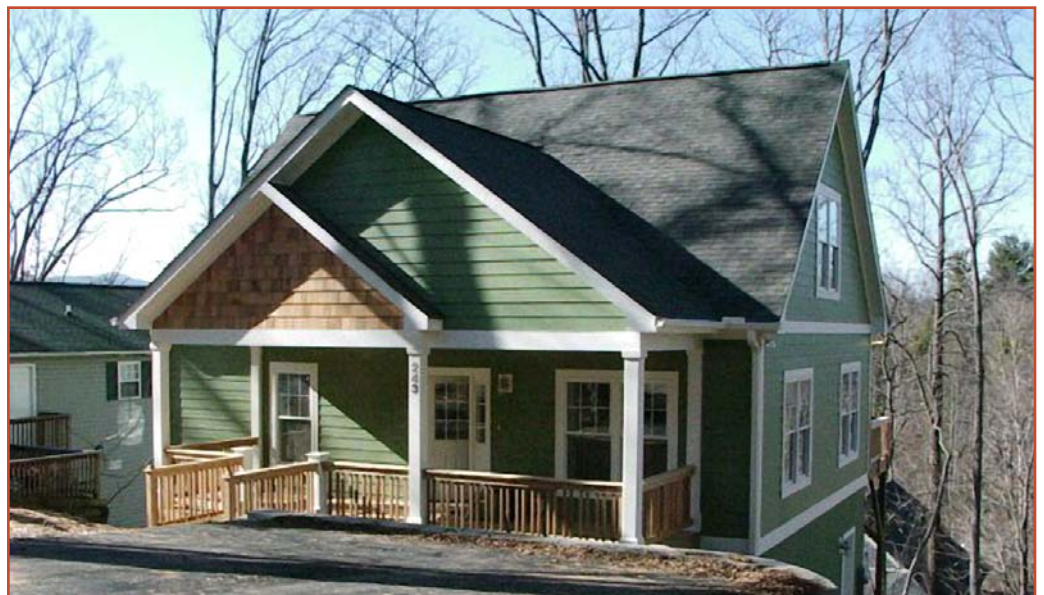
This Asheville home was the first modular home certified by the North Carolina HealthyBuilt Homes program.
